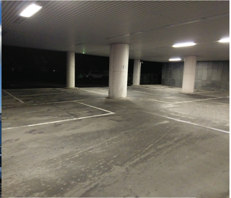
Figure 5: If on-street parking is free or cheap and readily available, nobody uses off-street parking. Source: Photo by Martina Hertel, Difu
