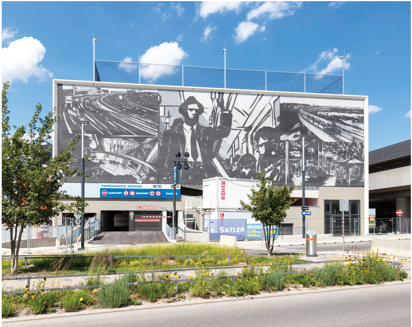
Figure 13: Shared Parking Garage in the Seestadt Aspern (City of Vienna, Austria). Source: © Daniel Hawelka
