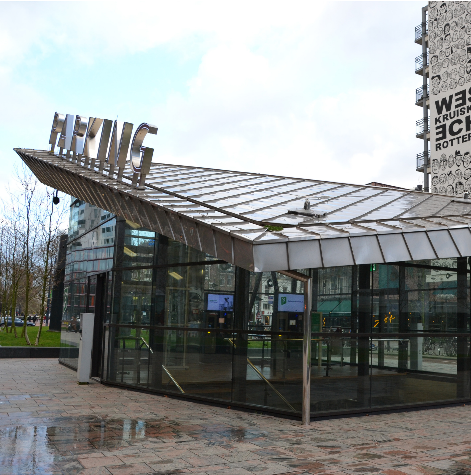
City of Rotterdam, New parking-facility © FGM / Harry Schiffer.
