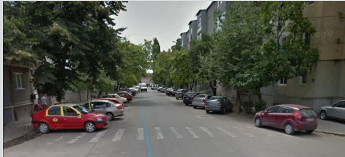
Before – illegal and abusive on-street parking Source: Google.com/maps/
