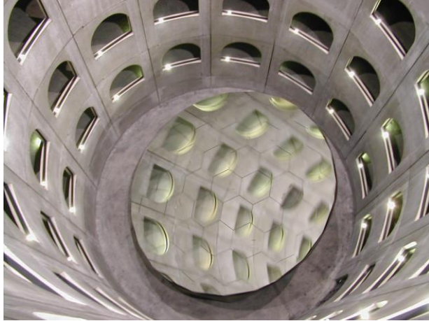
The kaleidoscope within the helical ramp of the Celestins underground parking structure
